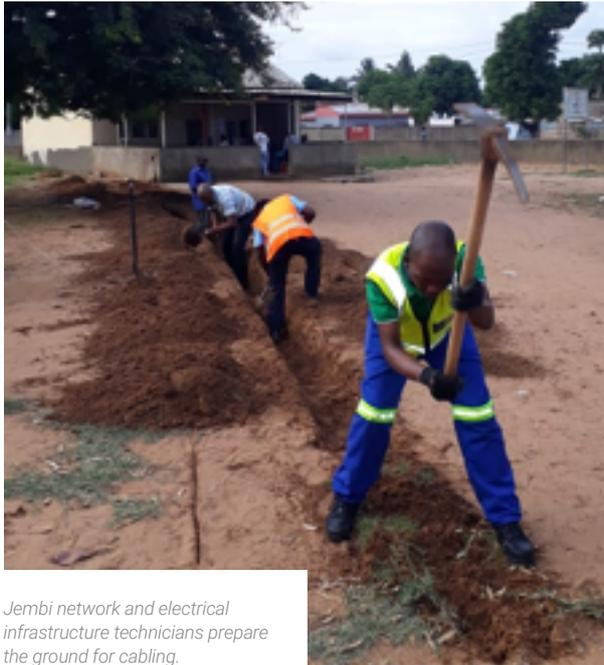
Jembi network and electrical infrastructure technicians prepare the ground for cabling.
